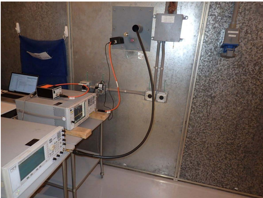
Section 21 RE System Verification Test Equipment (1 GHz - 6 GHz)
